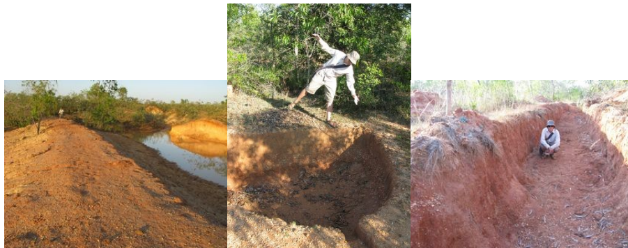
At the vertex of two dams by the mudpools #2 & #3; Kelly Hays tries to avoid a nasty fall into a water capture unit; Kelly Hays in a drainage trench near pool 2
